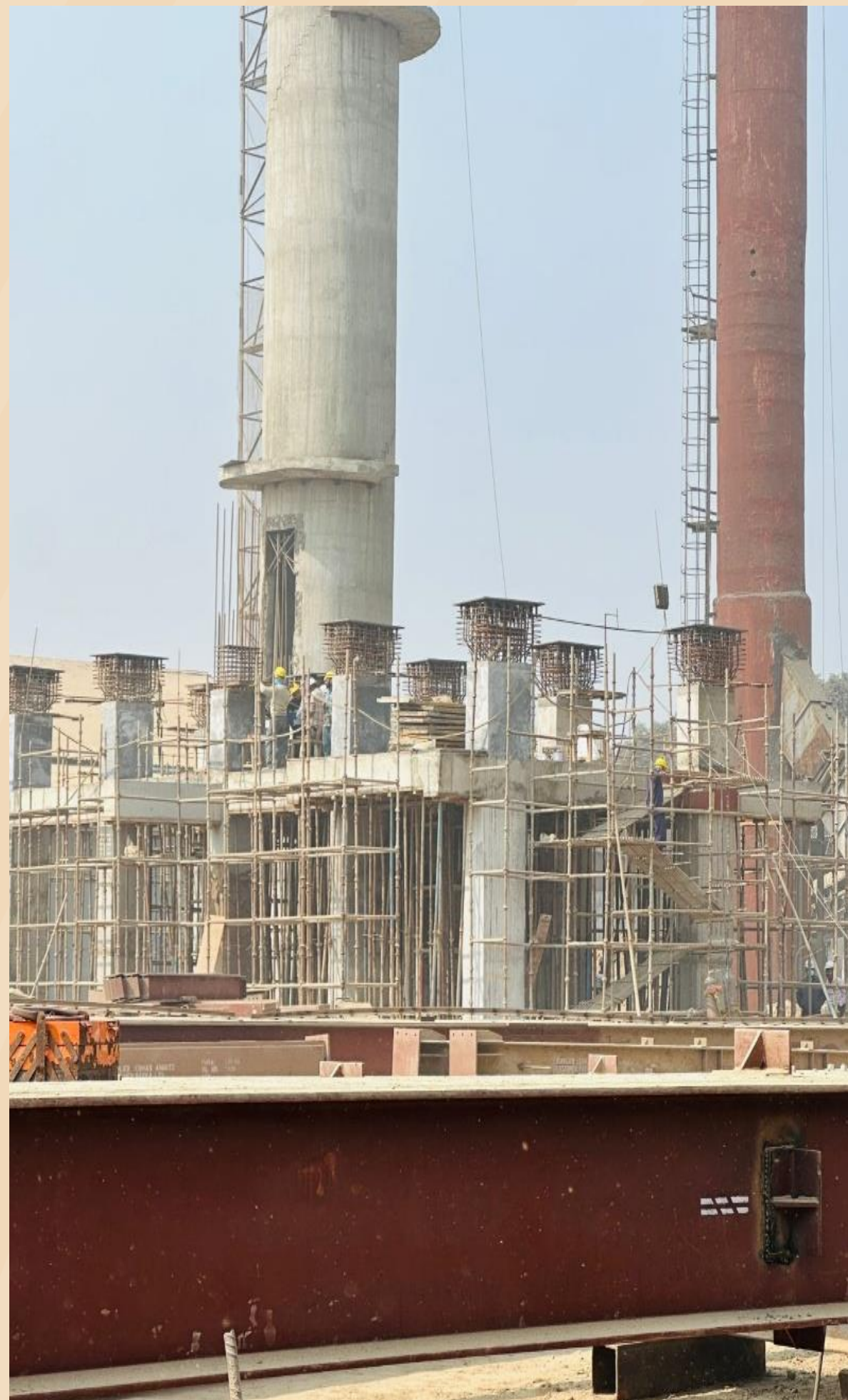
Recovery Boiler Upgrade
